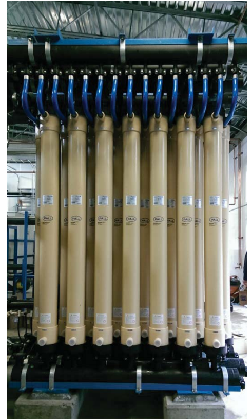
Newly installed Pall Membrane Filters
