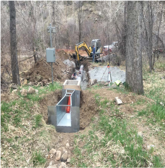
New Pipe line install
