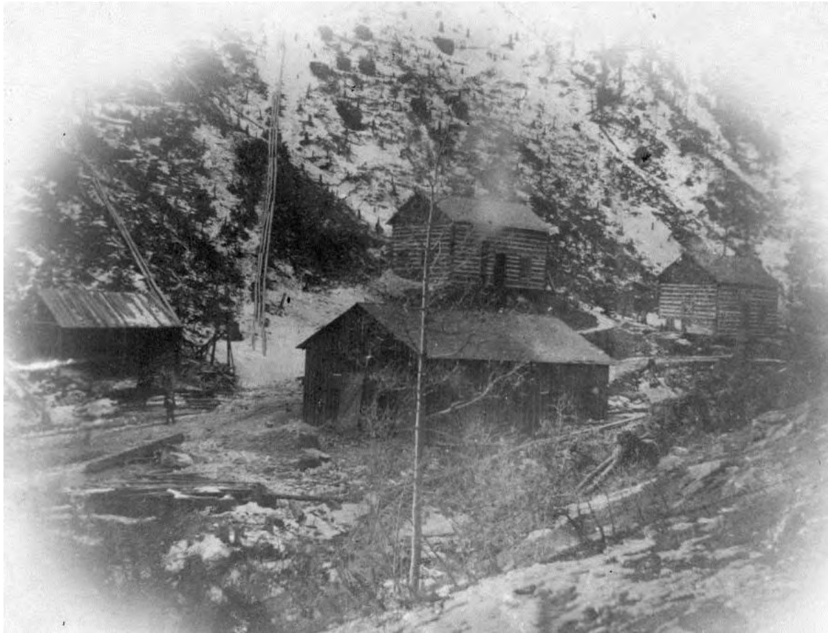
Figure 4.45: The view depicts two stamp mills, center and left, in lower Chase Gulch, 1861. The two other buildings in center-background and far right are log cabins. The stamp mills are deceiving in appearance, being simple and rectangular with low roofs. Denver Public Library X-2002.
