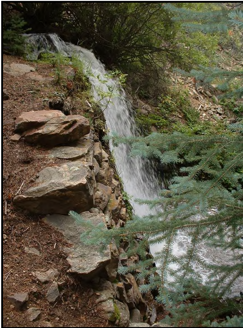
Figure 4.55: North profile of dam and Quartz Creek (5GL.2168). The dam face is at a batter, reclining leftward against the stream and soil creep. Workers chose large tabular rocks because they are heavy and fit together well.
