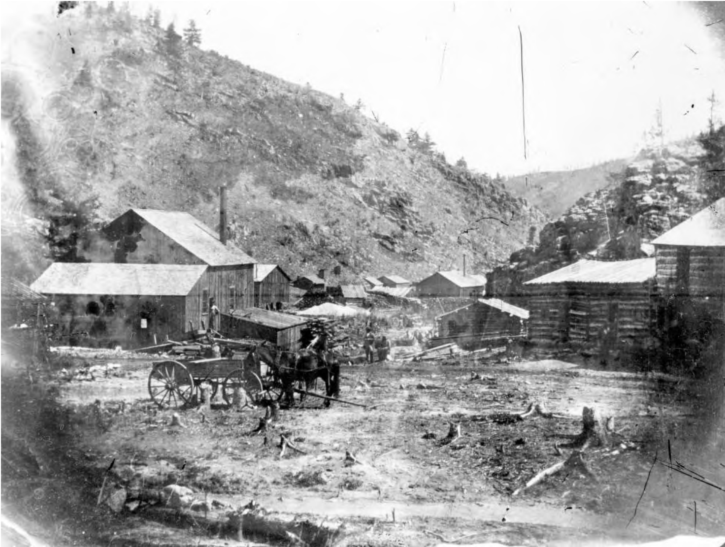
Figure 4.44: The 1860s photo depicts cabins and stamp mills lining the North Fork of Clear Creek, Black Hawk. The largest buildings at left and center-background with smokestacks are stamp mills with steam power. The mill discussed above was similar. Denver Public Library X-2034.
