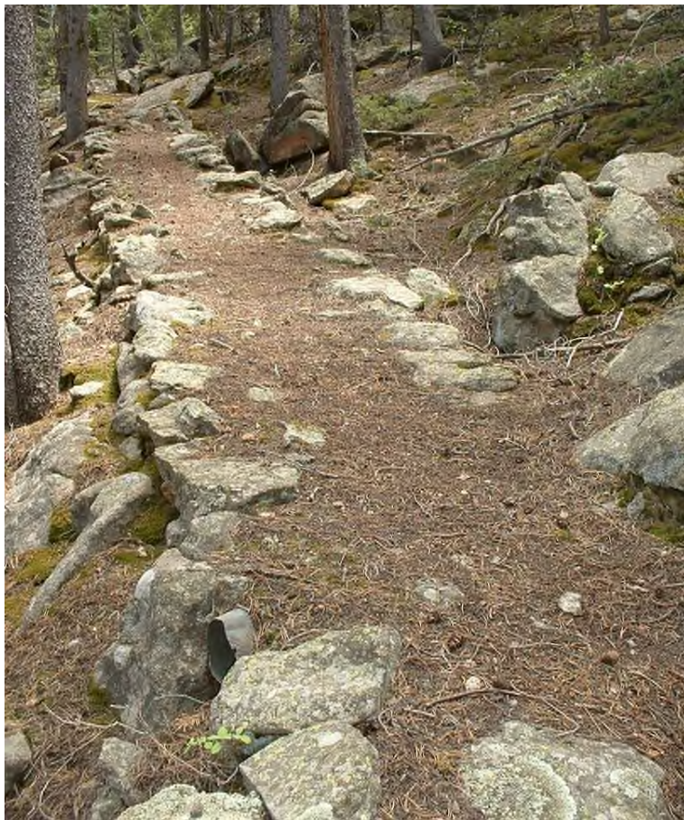
Figure 4.50: View south of Segment 4, 5GL.2161. The bed consists of sandy fill poured between two rock alignments, with a carefully depressed surface to cradle the pipeline. The left side was a gutter for storm runoff, drained through a stovepipe culvert visible at lower left.
