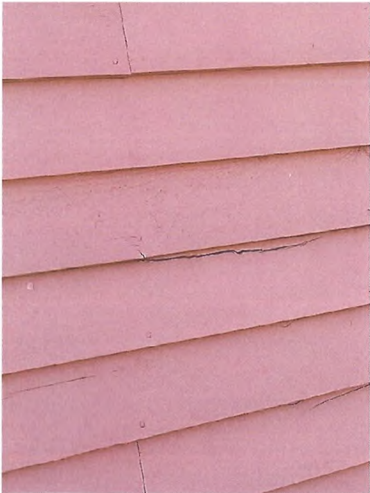
Cracks in siding – can they be caulked?
