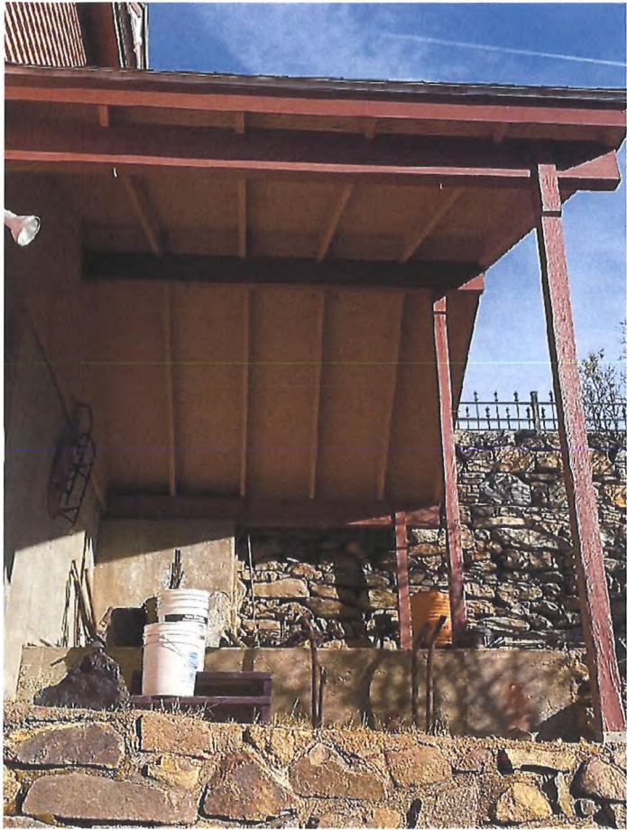
Bottom of porch roof is raw
