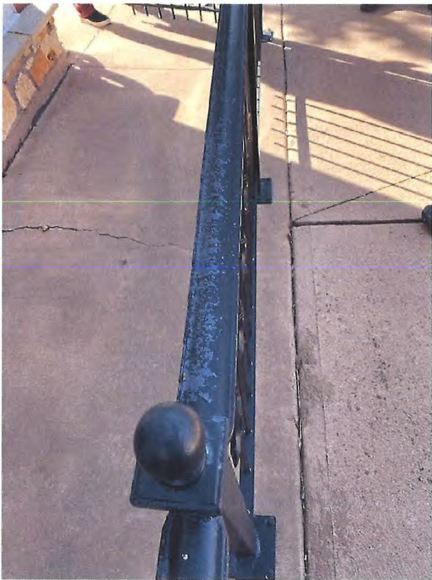
Metal railings in good shape but need to be painted
