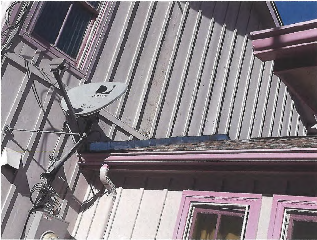
Raw flashing exposed
