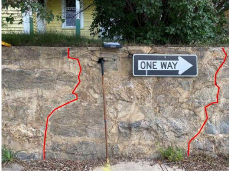
Figure 1. Many of the mortar head joints partially align, creating weaker connections between stones.
