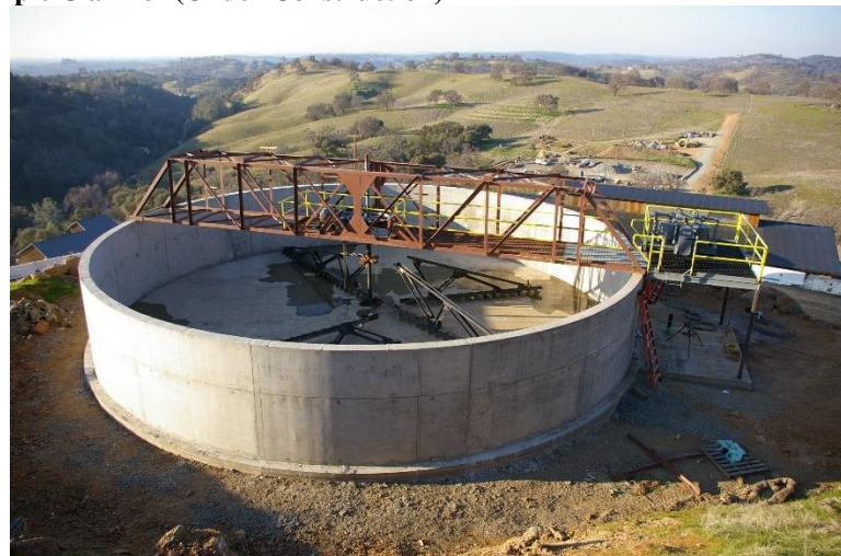
Figure 10 - Example Clarifier (Under Construction)
