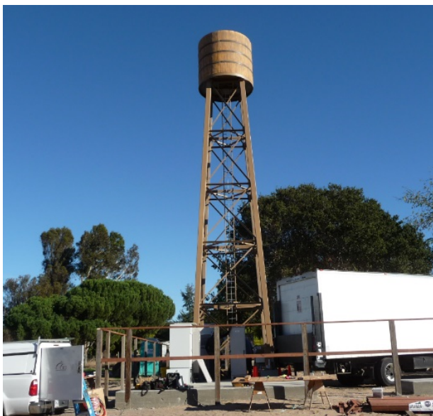
Example of faux water tower stealth design painted natural brown
